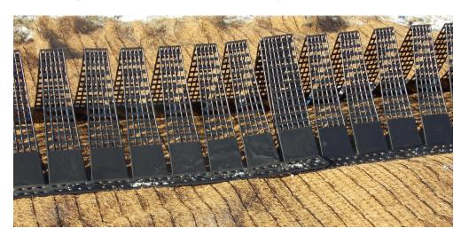
Enviro-Ridge reduces water velocity by distributing water over a wider area of the ditch bottom, facilitating sedimentation and revegetation. By dissipating energy and reducing flow velocity, Enviro-Ridge causes sediment to settle near the upslope side of each berm. In addition, its triangular configuration provides a protective shelter for newly emerging vegetation.
