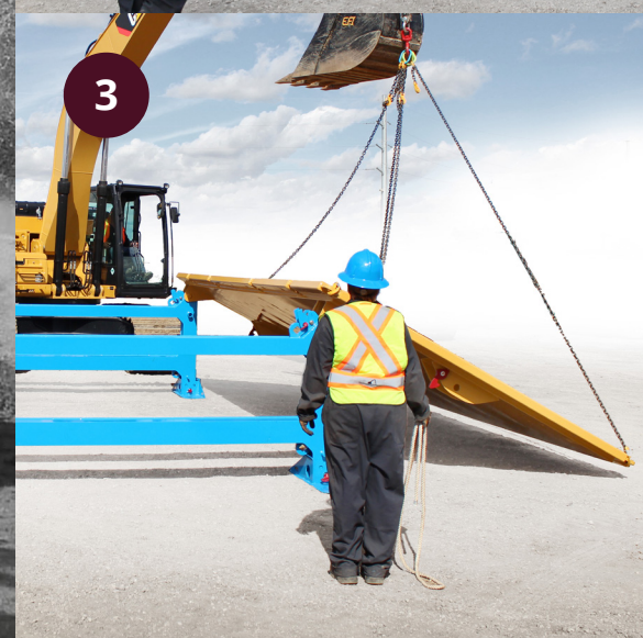
Gravity Locks engage locking the panels to struts before any worker enters the area to insert pins.
